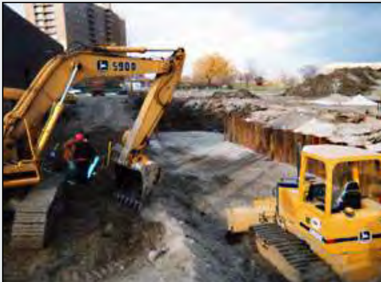
Excavation of Contaminated Soils (Photo Courtesy of MACTEC Engineering & Consulting, Inc.)
